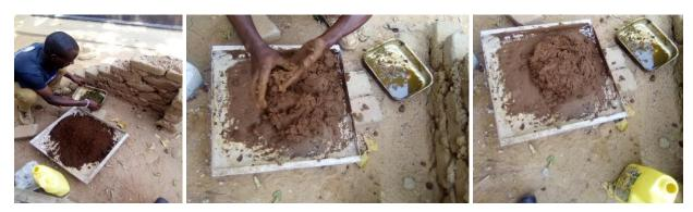
Figure 3: Mixing of cohesive soil with the cow dung
