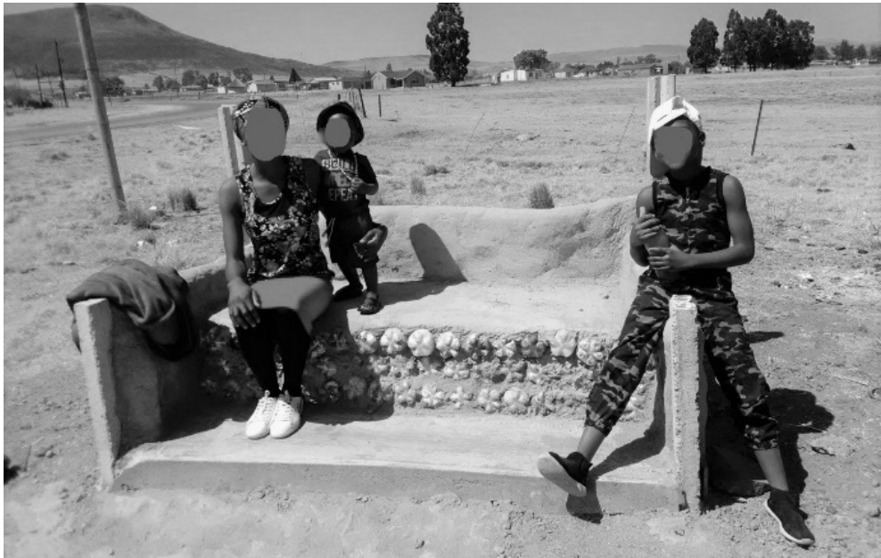
Figure 4: Bench made from eco-bricks (Preston, 2021, p. 209)
