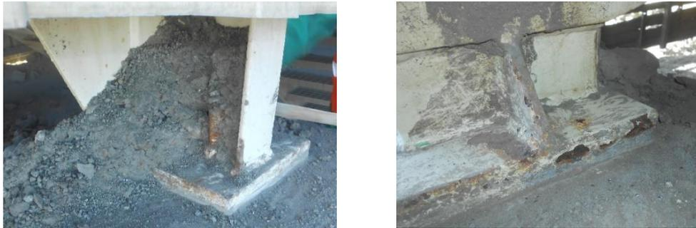
Figure 4 (left). Debris obscuring the metal surface
