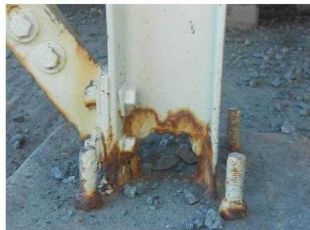
Figure 1. Localized corrosion that is causing the loss of load bearing capacity of a structural beam.
