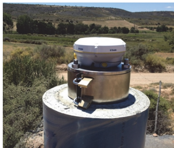
Figure 4. Receiver installed on stainless steel mount at Z031 with security band installed.
