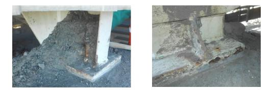
Figure 4 (left). Debris obscuring the metal surface Figure 5 (right). Corrosion damage evident only after debris has been removed.
