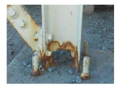
Figure 1. Localized corrosion that is causing the loss of load bearing capacity of a structural beam. How long will it last?
