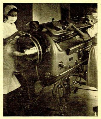
Fig. 1. The modern tank respirator (Drager) with the dome being placed in position.
