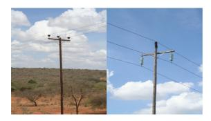
Figure 1a & b. 1a (on the left) shows the typical "T-structure" which poses an electrocution risk to birds perching on the cross arm. 1b shows the "inverted T" pole structure which is safer for perching birds since the outer conductors are suspended below the cross arm out of reach of birds.
