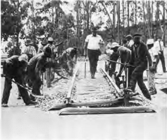
The construction of the Track
