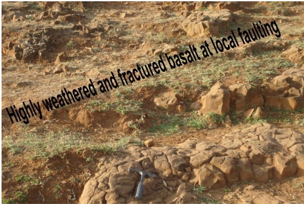
Figure 13: Highly weathered and fractured basalt at local faulting of the selected irrigation fields in the study area.
