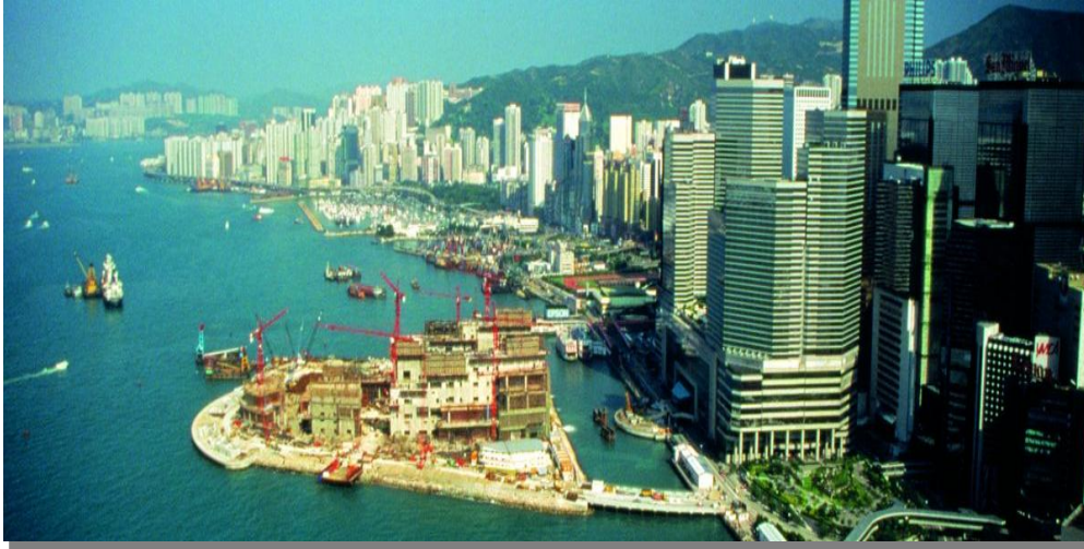
Figure 2: 1997 Infrastructure Expansion Milestone
