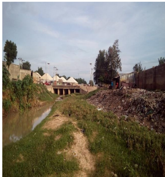
Plate 3. Refuse dump in a River Channel
