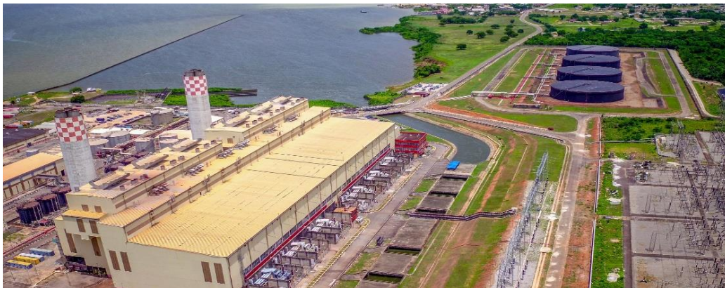
Figure 1: Aerial view of Egbin power plant (Partners, 2018).
