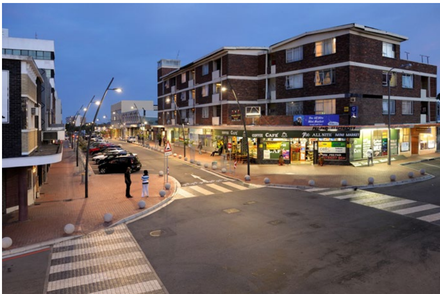
Figure 4: A lively section of the upgraded Parliament Street
