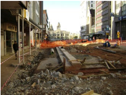
Figure 2: Upgrading of Govan Mbeki Avenue
