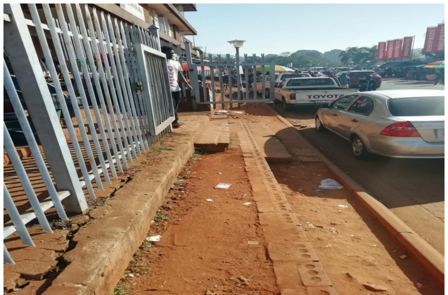
Figure 5: Fenced pavement posing a safety threat to pedestrians Source: Image taken by Tsoriyo, 2020
