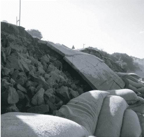
Plate 1: Damage to the coast under marginally high seas (Umdloti Beach - June 2011). (Source: Oceanographic Research Institute, Durban)
