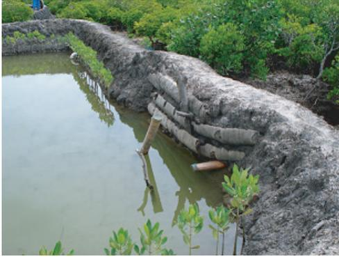
Figure 2. A pond at Majaoni showing the PVC standpipe to drain the pond and the overflow pipe that allowed water exchange at spring high tides and maintained the water level.
