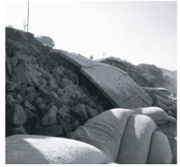
Plate 1: Damage to the coast under marginally high seas (Umdloti Beach - June 2011). (Source: Oceanographic Research Institute, Durban)
