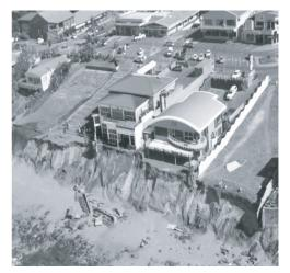
Plate 2: Damage to buildings as a result of the 2007 extreme weather event (Ballito, KZN North Coast – March 2007). (Source: Simon Bundy)
