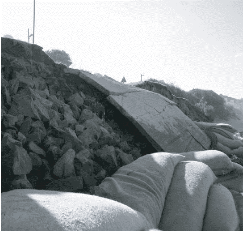
Plate 1: Damage to the coast under marginally high seas (Umdlotti Beach - June 2011). (Source: Oceanographic Research Institute, Durban)
