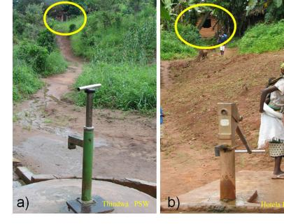
Figure 4 Protected shallow well (a) and borehole (b) located downhill from latrines/ toilets
