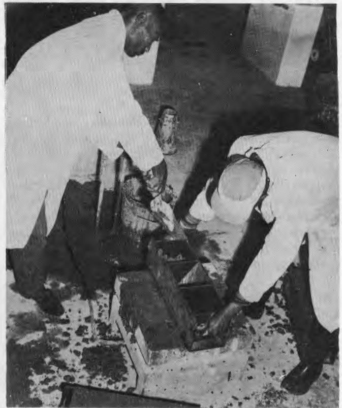
Picture 2 — Cubic test specimens of concrete being moulded.
